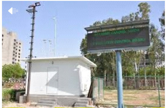
Continuous Ambient Air Quality Monitoring System
