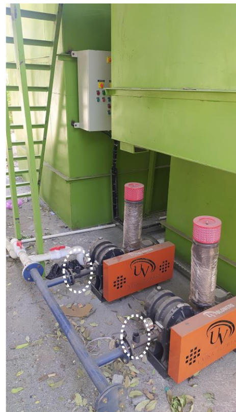
Figure 12 The missing valves of a yet to be commissioned greywater treatment facility located in a park in Sinnar
