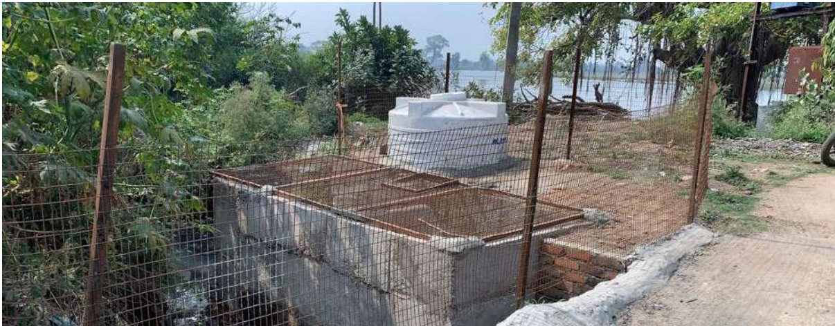
Figure 37: Completed project site
