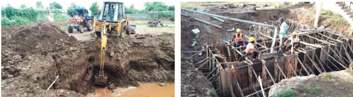
Figure 28: Scaffolding to address landslide and waterlogging on site
