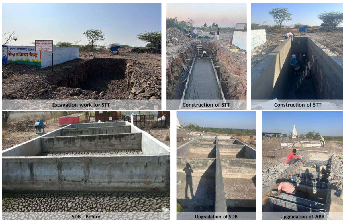
Figure 18: Construction work of FSTP refurbishment at Indapur
