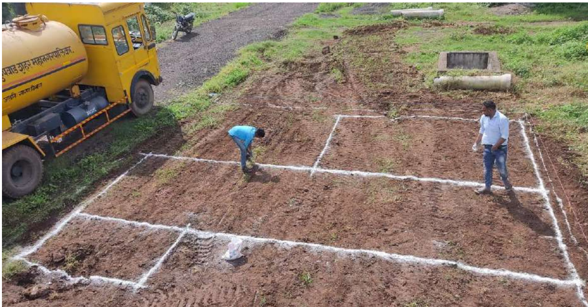
Figure 22: Lineout for Co Treatment Units
