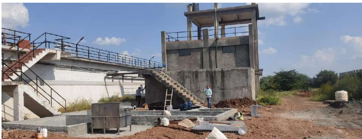
Figure 24: Mid-construction stage at Co treatment Plant
