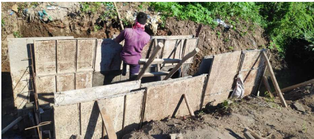
Figure 36: Construction activities on drain in Bhiwapur
