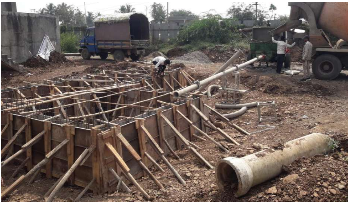
Figure 23: Construction of the co-treatment units at the STP
