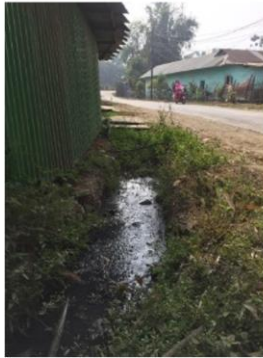
Unlined, open drains
