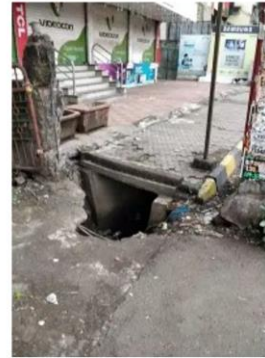
Lined, covered drains
